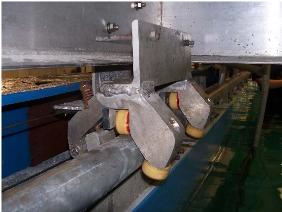
Figure 7. Complete Truck Installed On Carriage
