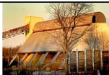
Old Town Fuel and Fiber is run out of a converted paper mill.
