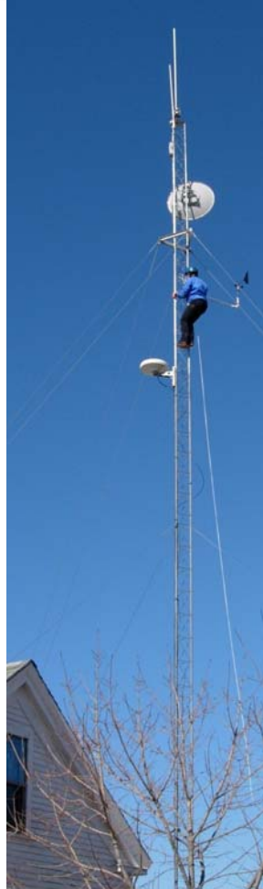
Levi mounts an anemometer on the communications tower on Matinicus
